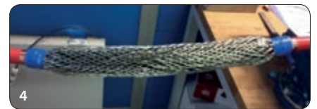
4 The metal shield is rebuilt
