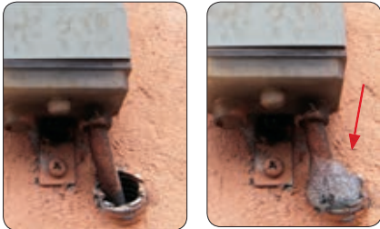
Corrugated pipe entry protection
