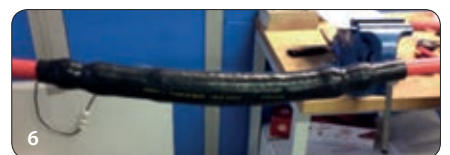
6 The joint is ready and can be used immediately
