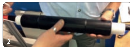
2 Position at the centre of the connection
