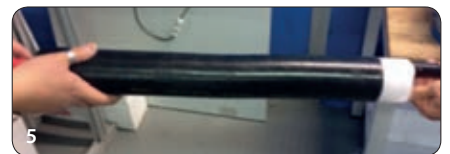
5 The outer protective sheath is positioned and installed
